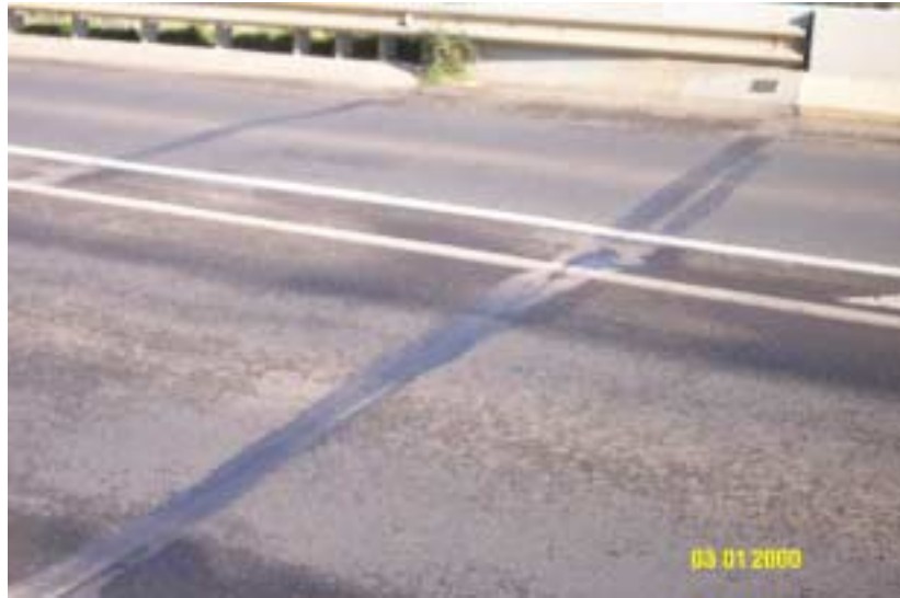
Figure 14: Approach Pavement Crack and Joint Filling
