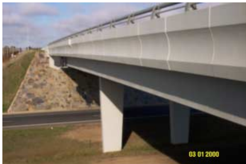
Figure 9: Bridge Deck View
