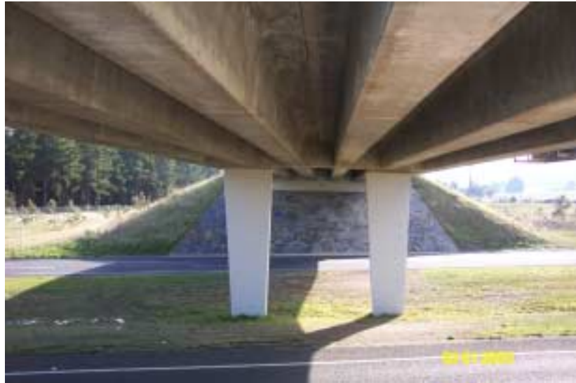
Figure 10: Underneath View Showing Central Pier
