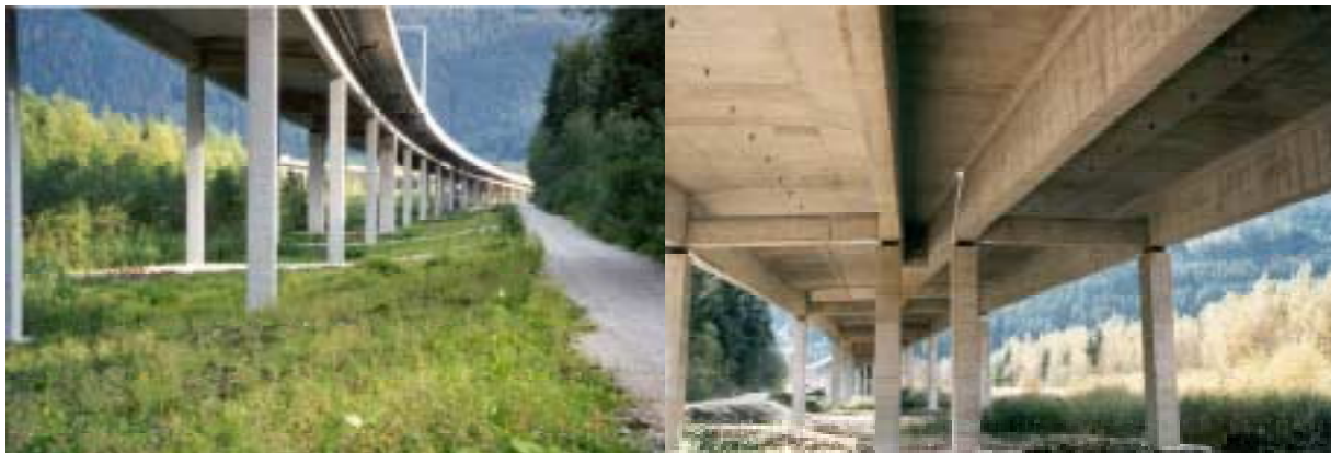
Figure 1. KS7 Selzthal (Austria) – Transition from double Tee to quadruple Tee-beam.
