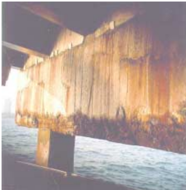
Figure 7: Cracking along the upper reinforcing bars and honeycombing at the bottom edge of crosshead
