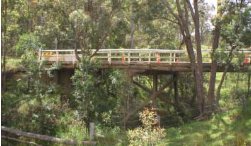
Figure 4: Side elevation of Hunter Valley bridge
