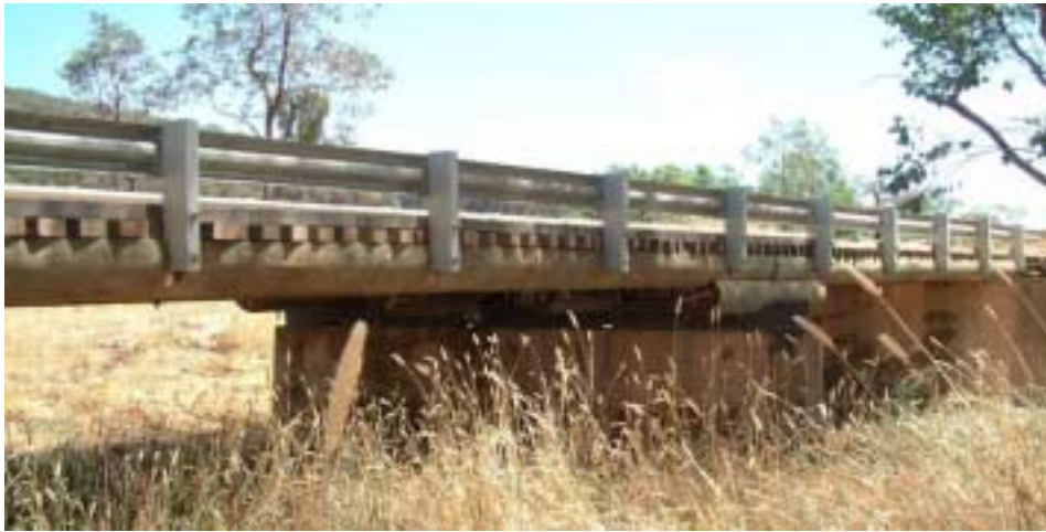
Figure 2: Side view of Cabonne bridge
