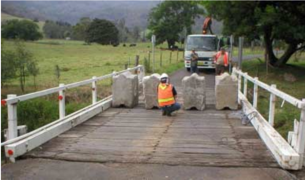
Figure 6: Testing with mass applied at mid span
